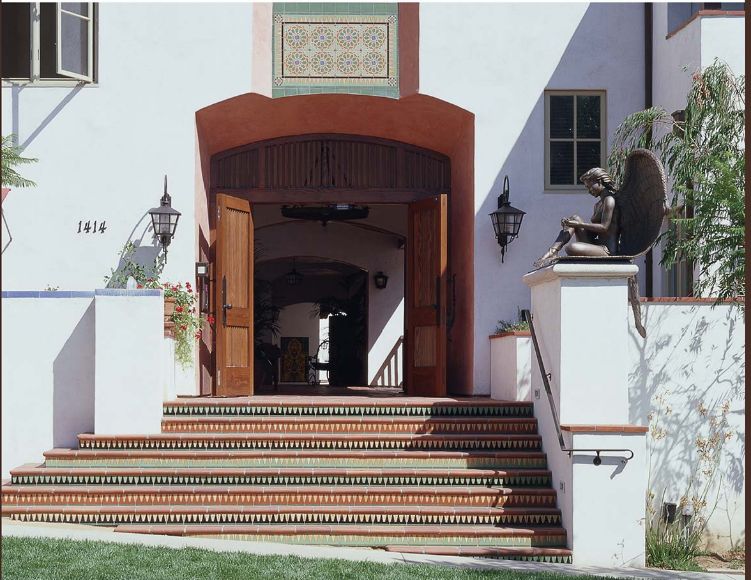
7 FOUNTAINS WEST HOLLYWOOD, CALIFORNIA CUSTOM MURALS, FLOOR TILE, STAIR RISERS & FOUNTAINS.
